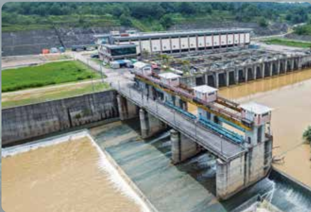
Semantan Raw Water Intake
