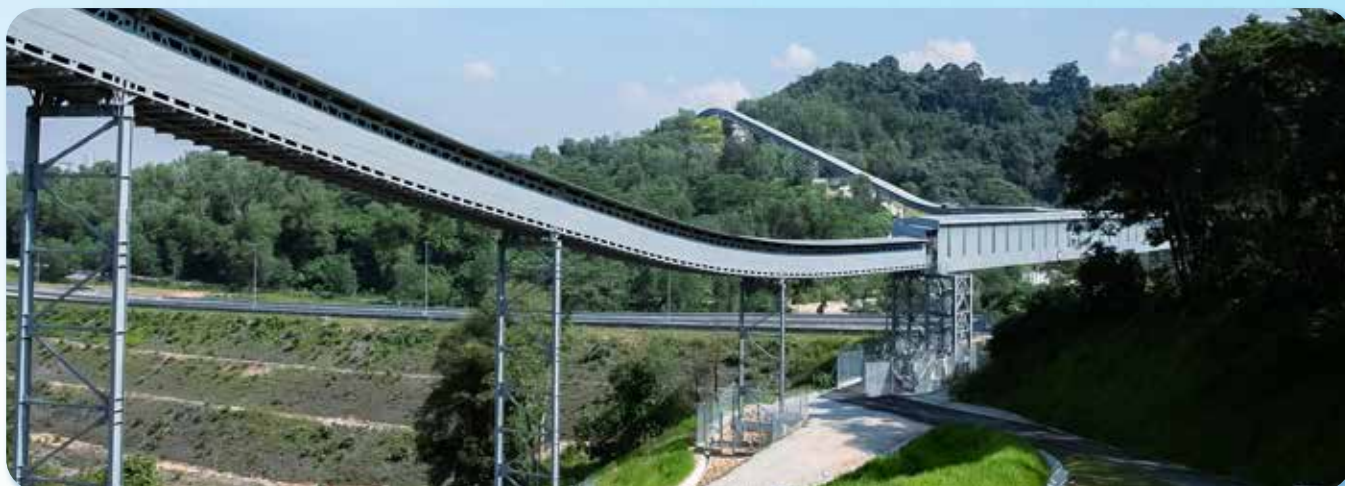
Langat 2 Phase 1 & 2 Residual Pipe Conveyer System
