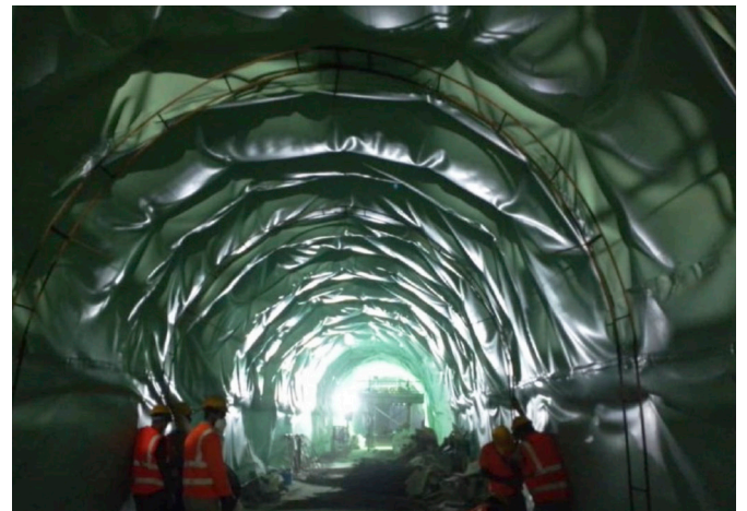
Application of synthetic (PVC) waterproofing membrane
