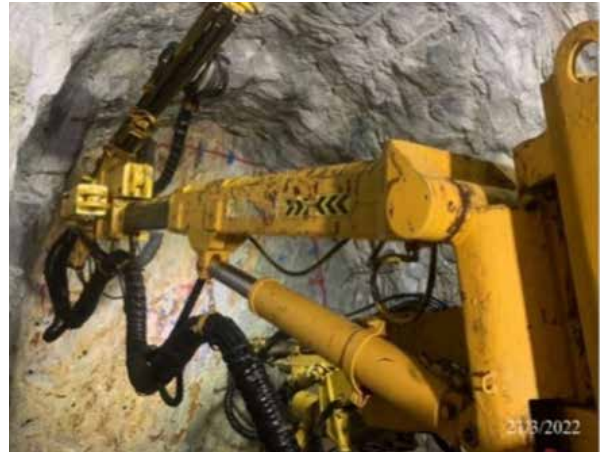
Figure 4: Marking and Blasting during excavation of work
