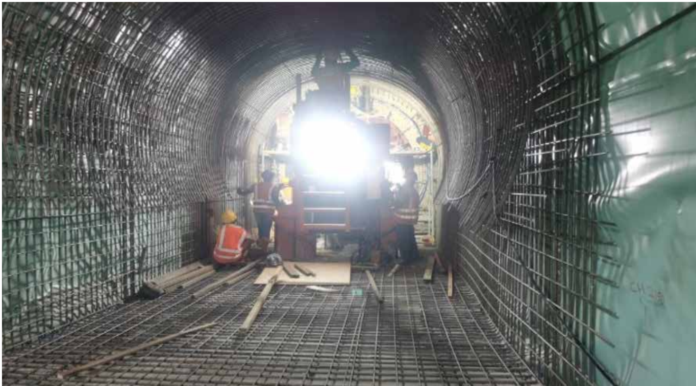
Figure 5: Installation of rebar concrete lining in progress
