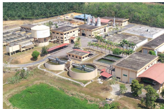
○ Overview of Sawah Raja WTP Phase 1 & Phase 2, Chemicals Buildings, Clear Water Tank, Booster Station and Residual Treatment Facilities
