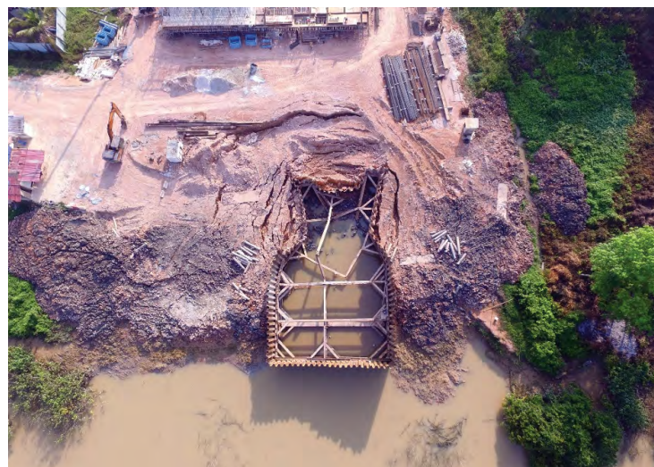
Original construction using Cofferdam method
