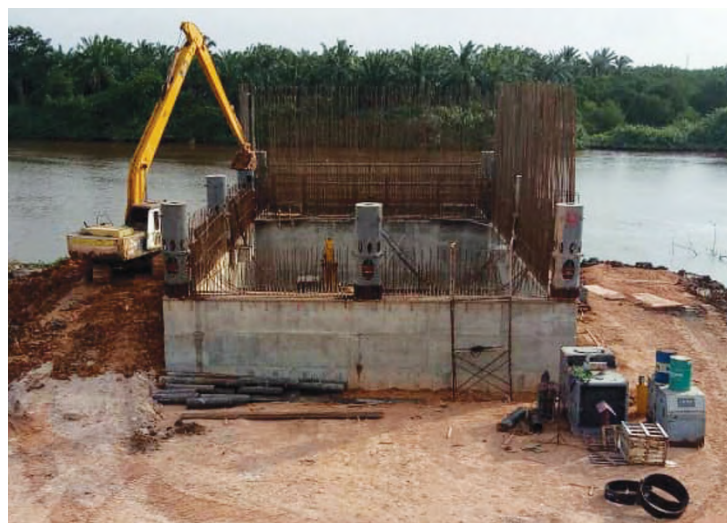
Construction of Intake Using Caisson Method
