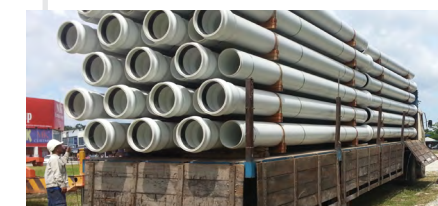
Unloading of MuPVC pipes at Batu Pahat site
