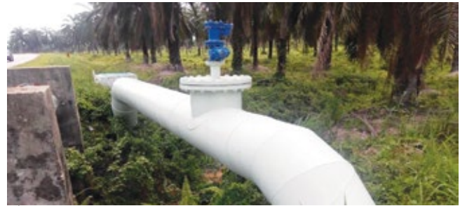
700mm Dia. Mild Steel Pipeline
