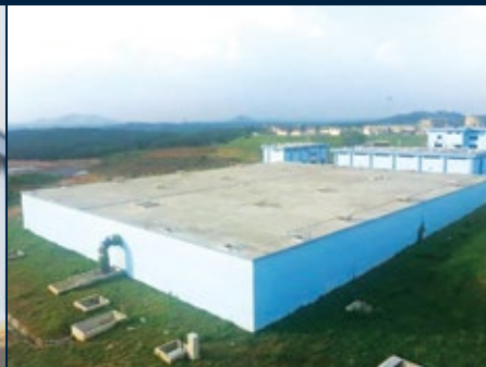
Contact and Clear Water Tank
