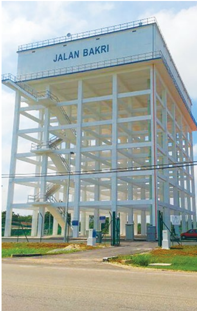
3.5 ML Jalan Bakri Reservoir
