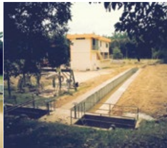
Raw Water Intake Plant at Kg Jambu Lapan
