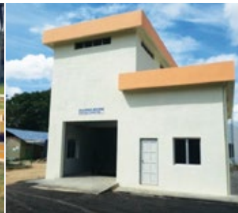
Residual Holding Tank & Thickener Tank
