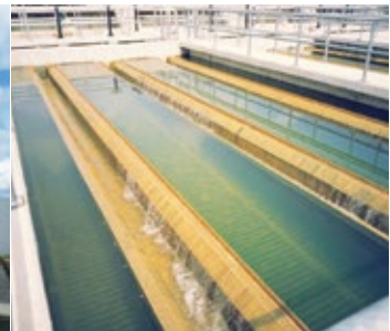
Thickened Residual Building
