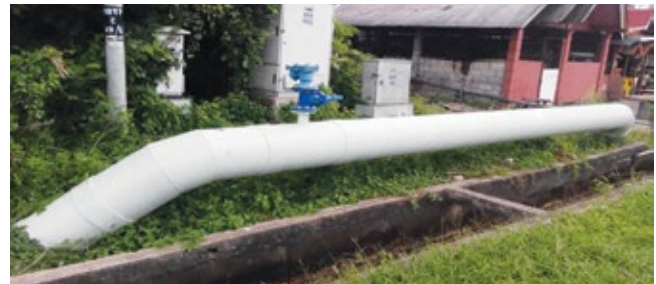
450mm Dia. Mild Steel Pipeline
